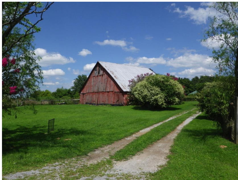
Figure 44. R-11, facing north.
