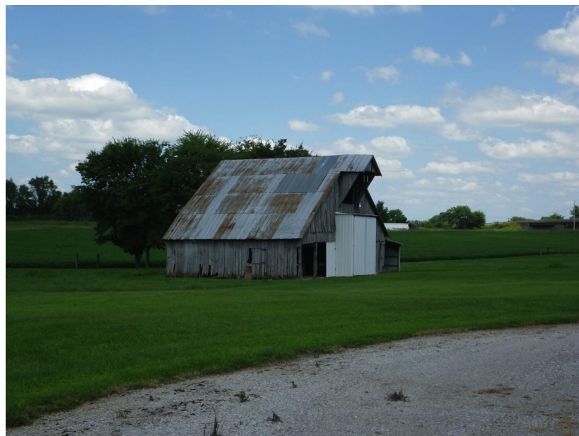
Figure 42. R-9, facing north.
