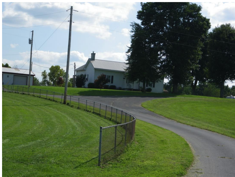
Figure 46. R-13, facing southwest.
