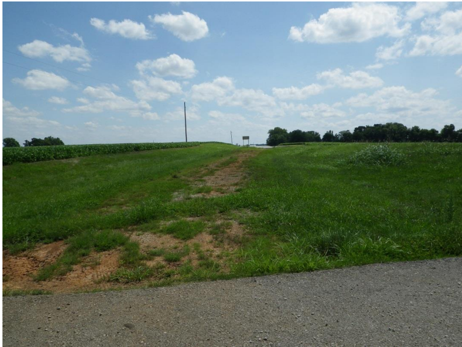
Figure 35. Remnant of Old SR 345 (Beverly South Rd) near Intersection of SR 345 (Palmyra), facing south.
