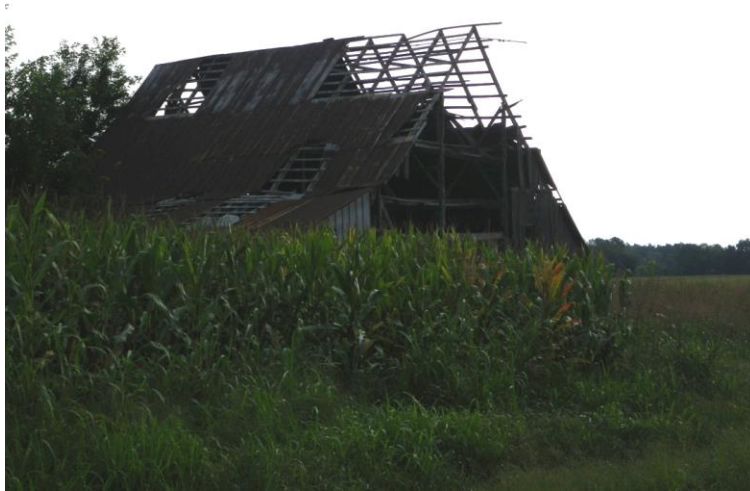
Figure 49. R-16, facing northeast.
