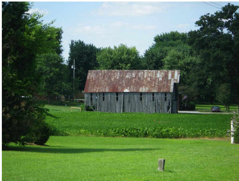
Figure 48. R-15, facing north.
