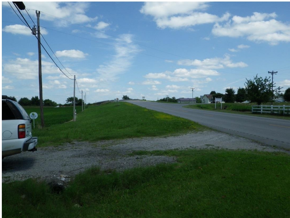
Figure 33. KY 107/KY 345 overpass of I-24, and KY 107 intersection with KY 345 (upper right), facing north.
